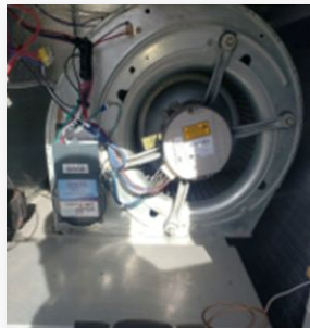
Ionizer units installed on HVAC
